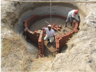
Constructing a Bio Gas Oven at Punanawa – 23 Nov 2010
